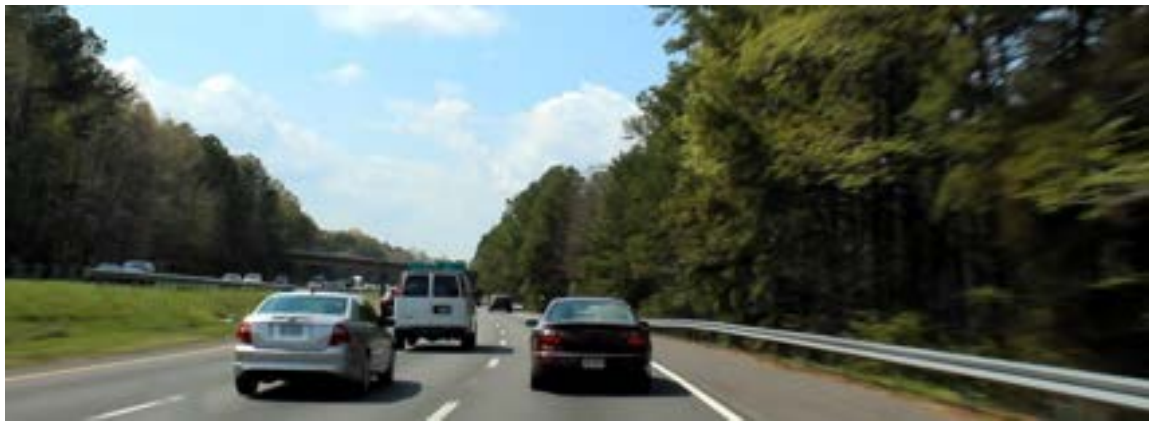
Figure 29. Example of a control DCZ on a freeway.
